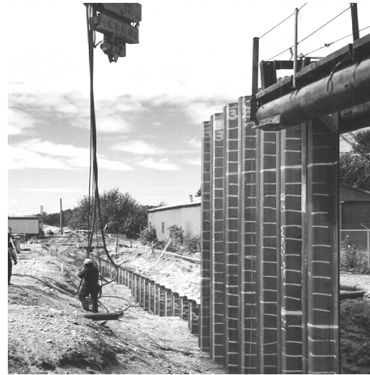
Photo 1. Driving WEZ-95 sheet pile using driving frame.
