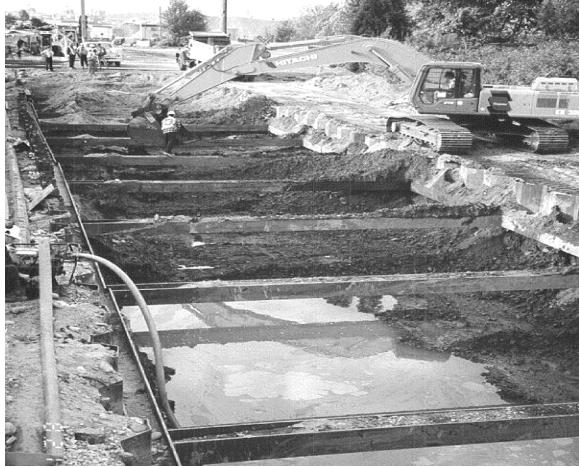
Photo 2. Excavation with secondary sheet piling shoring.
