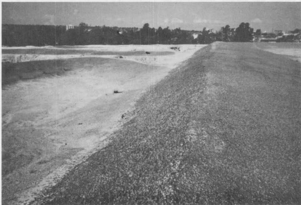
Fig. 6—Appearance of paddock walls protected against wind and water erosion by a single layer of 19 mm of crushed-stone chips. Photograph taken two years after laying
