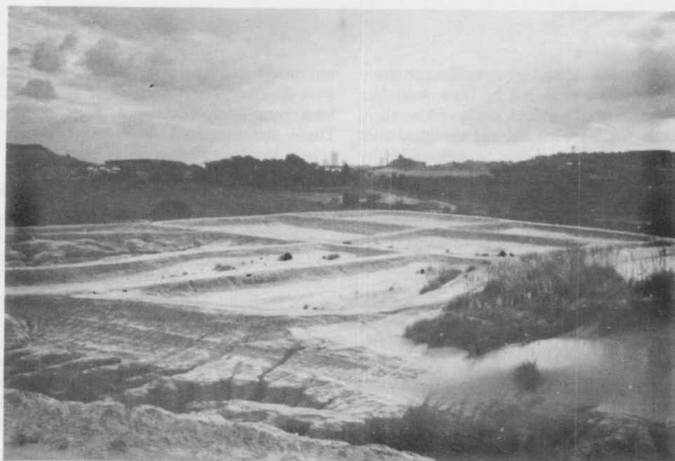
Fig. 3—Abandoned tailings dam provided with crest and dividing walls
